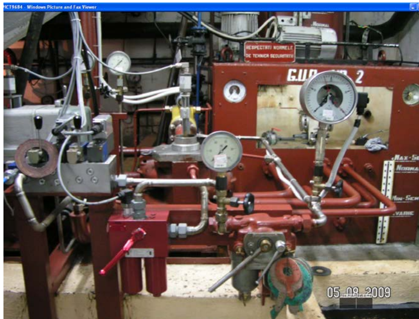
Fig.2 Modernizations works The Oil pressure group
