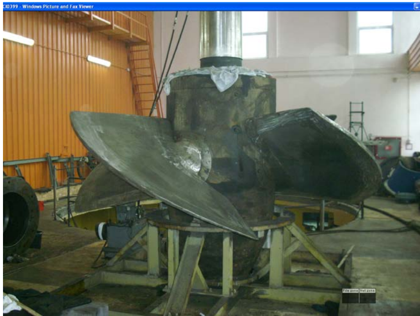
Fig.1. Kaplan rotor of turbine – removed on the platform
